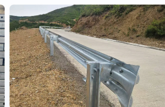
W beam galvanized guardrail
