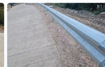
TIS 248-2531 W beam galvanized guardrail
